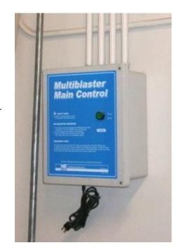
additional Hydroblaster's as needed, bringing them on line until all are in use. When all Hydroblaster's are in use, the remote location enunciator lights will remain on (without blinking). During a period of non-use, at the activating station, system automatically turns off the Hydroblaster assigned to that station. This automatic "shut down timer" eliminates needless wear and tear on the Hydroblaster's.
