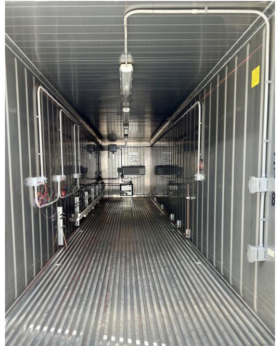
Electrical and plumbing installed prior to equipment installation
